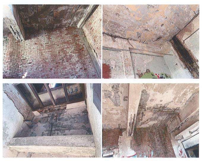
Because this building's use did not expose the structure to a high degree of chlorides over time, the level of corrosion is quite limited and minor in nature. Its repair would consist of the cleaning of corroded reinforcing steel and patching the concrete. This is a fairly commonplace repair with reinforced concrete structures of this age.
