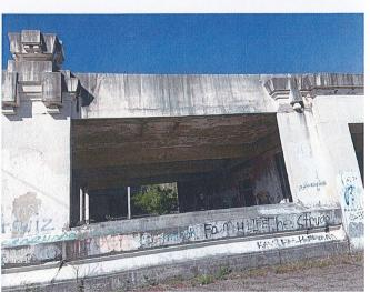
Additionally, there are substantial concrete walls as part of the reinforced concrete frame for this building which would give it substantial lateral system capabilities well over and above anything required by modern building code.
